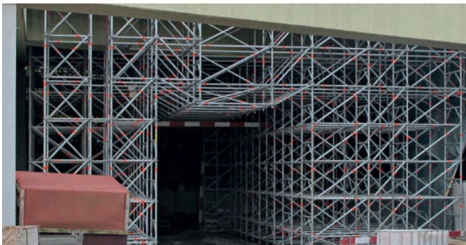
Bridging structure/passageway in shoring scaffolding using standard Allround Scaffolding material.
