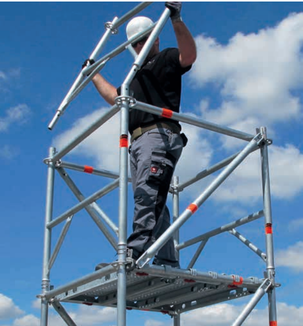
Safer upright assembly thanks to integrated and advancing side protection
