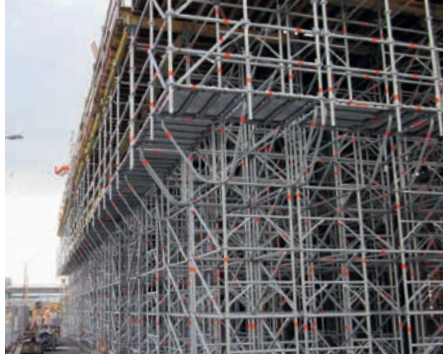
Attachment of bracket deck surfaces at edge.
