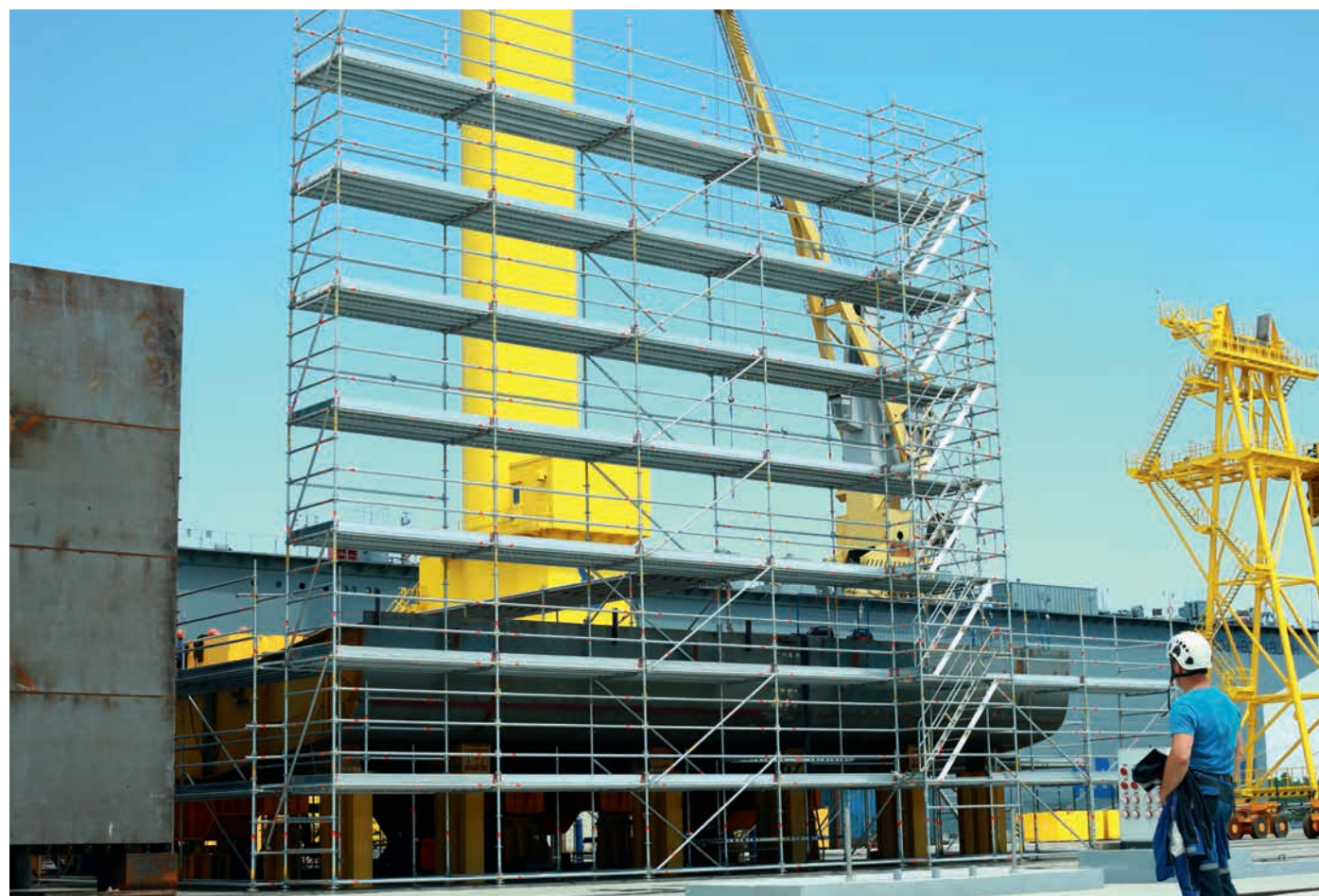
Reduction of fire risk in both simple and complex scaffolding using steel toe boards
