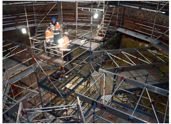
Bridging with Aluminium FlexBeam for scaffolding inside a boiler
