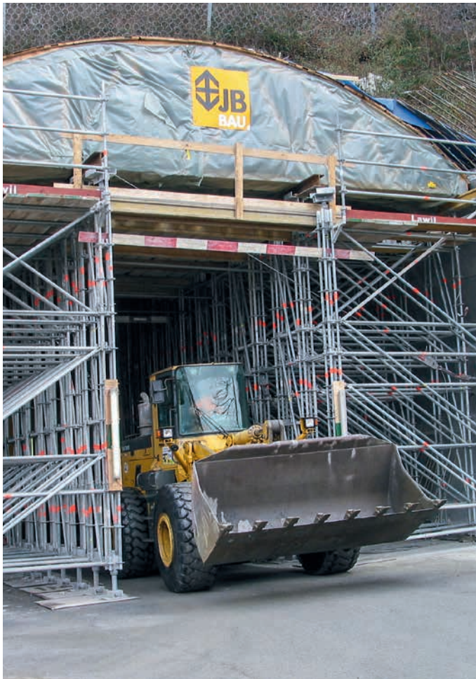
Shoring made using Allround Scaffolding with combined standards and a passage opening for vehicles
