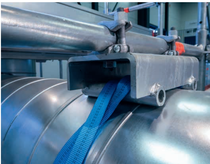
Suspended scaffolding adapter on pipeline
