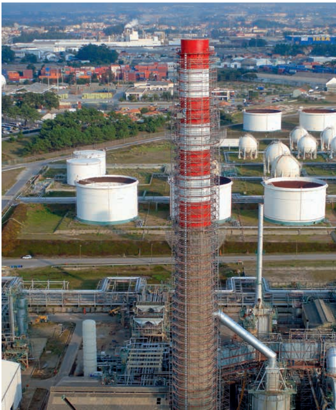
Circular scaffolding with Allround Scaffolding on a refinery column
