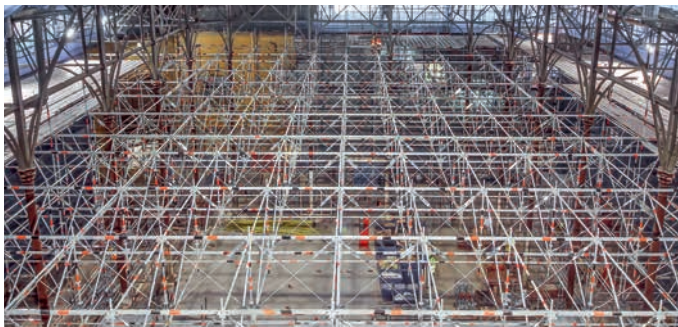
Birdcage scaffolding with Allround FW System inside a building – the floor area remains free, allowing normal work to continue
