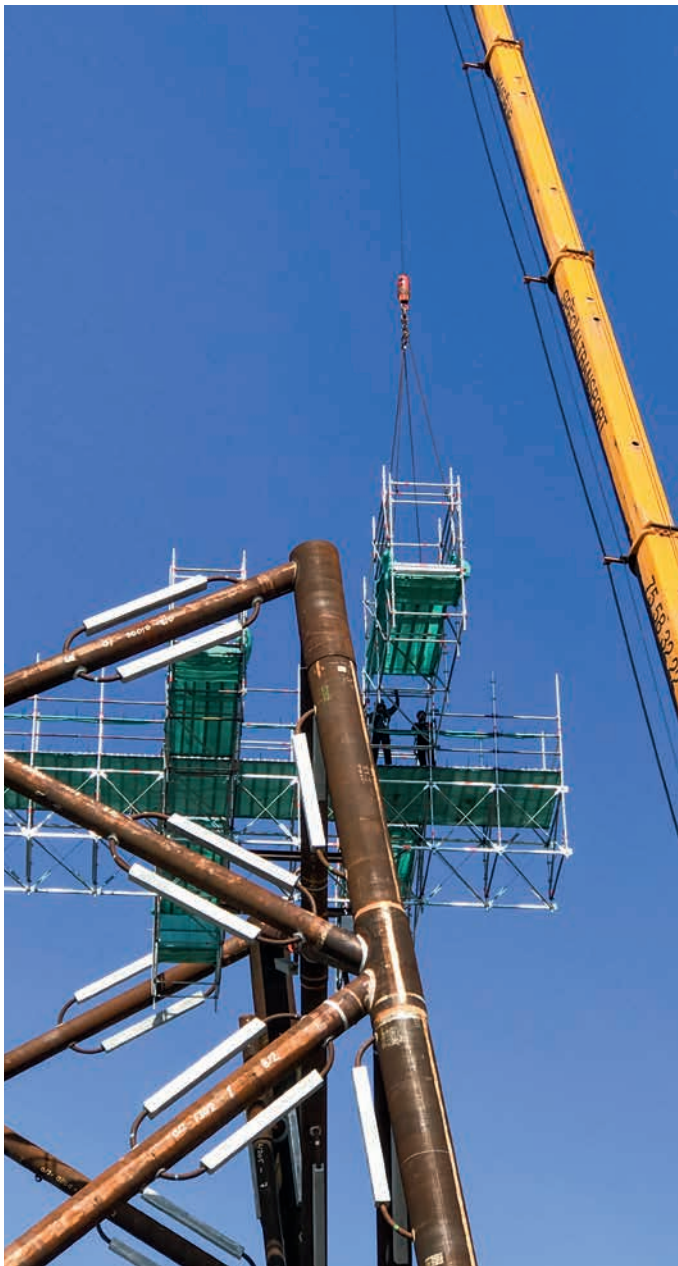
Self-supporting suspended scaffolding preassembled on the ground with the Allround FW System
