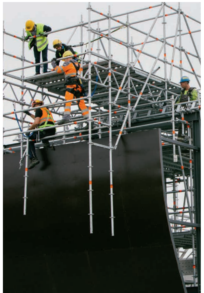
Assembly of mobile suspended scaffolding on rails
