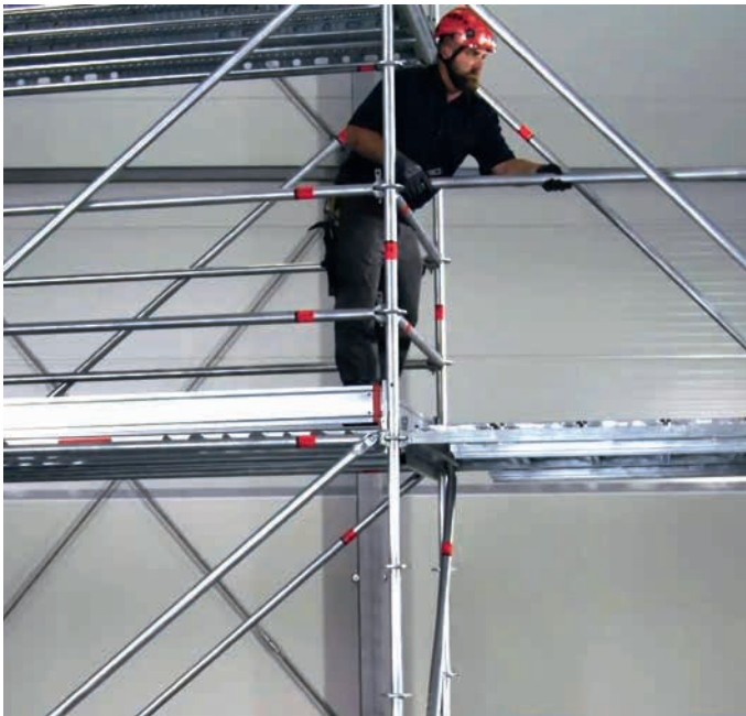
Allround Scaffolding using the cantilever method
