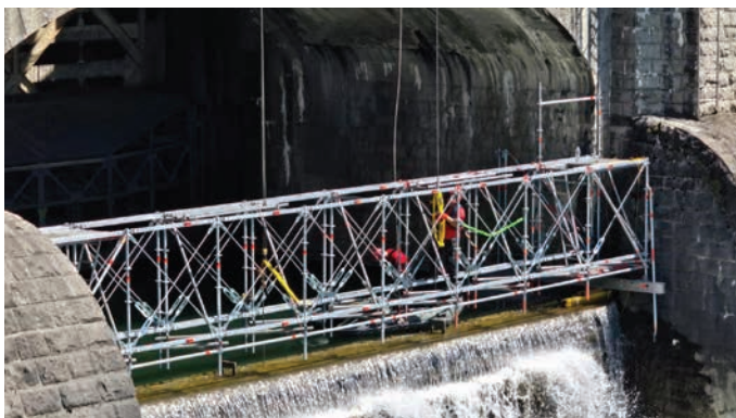
Mobile suspended work platform with Allround FW System
