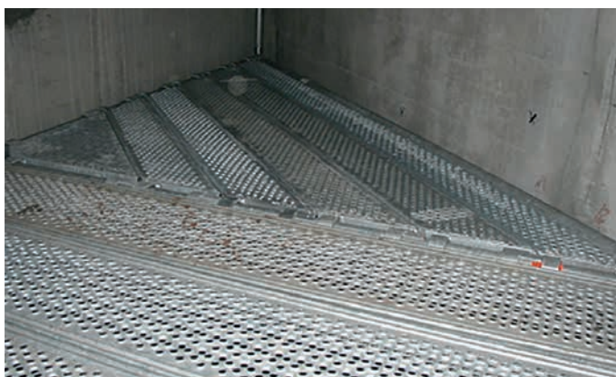
Triangular and trapezoidal decks for level decking of 45-degree inner corners
