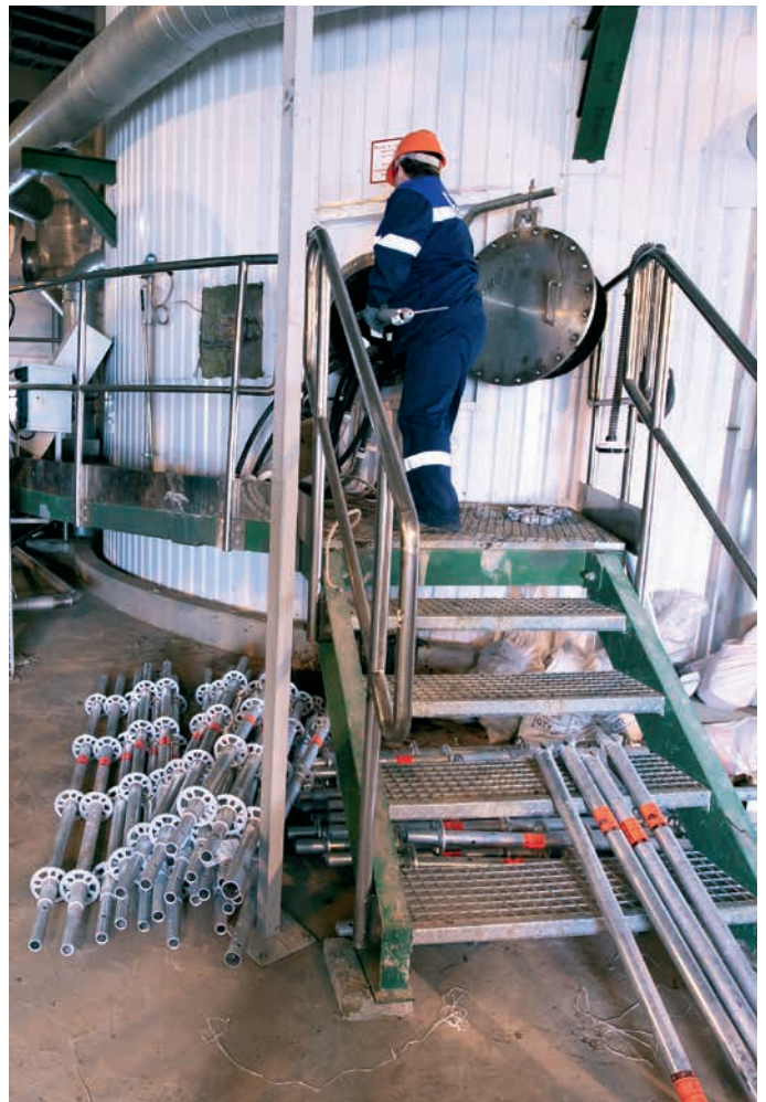
Compact and lightweight parts permit transport of material through narrow manholes
