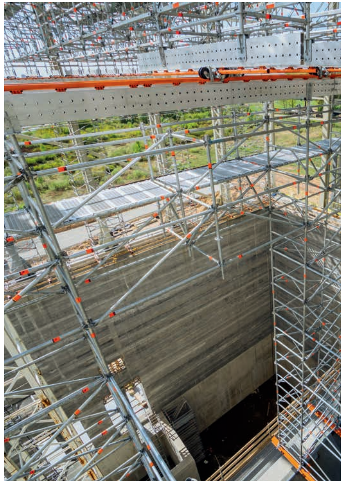
Shoring TG 60 in combination with the Aluminium FlexBeam and the Allround FW System when building a new industrial plant
