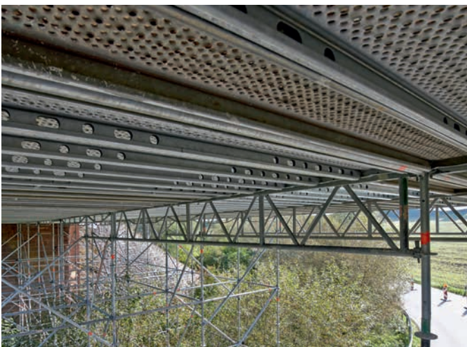
Bridging using Allround system lattice beams
