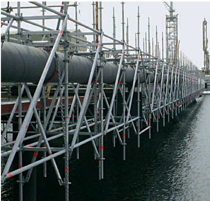
Suspended scaffolding on pipeline – attached using chains with suspended scaffolding adapters
