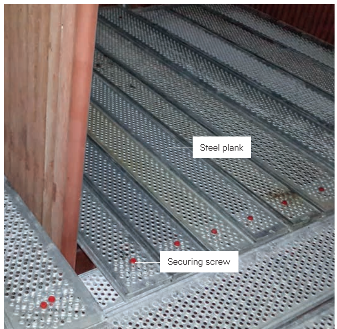
Steel planks, secured with long locking screws (red), on steel decks
