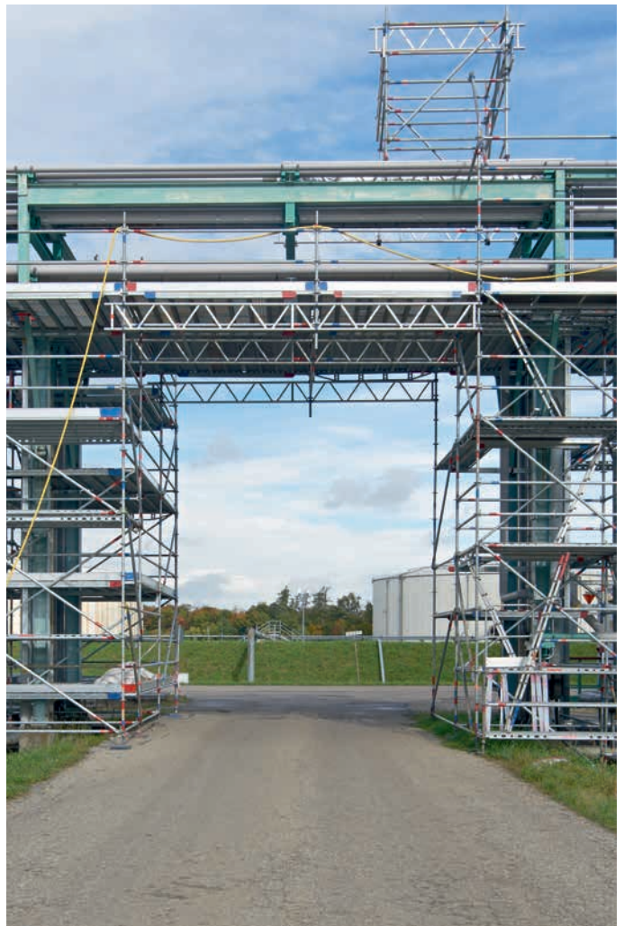
Bridging with Steel System Lattice Beams 450 LW from the Layher accessories range
