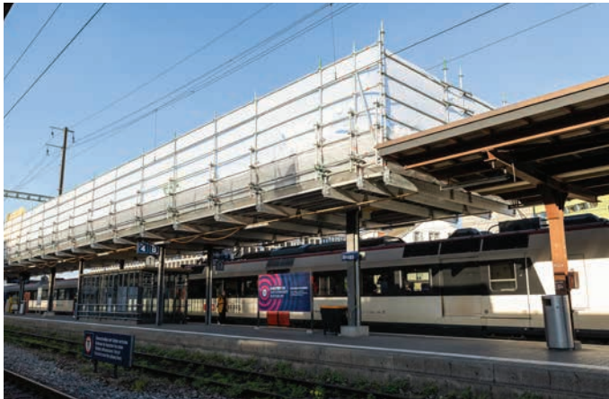
Projected suspended scaffolding with protective wall
