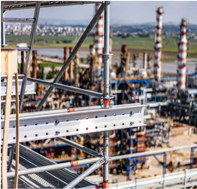
Work scaffolding suspended on Aluminium TwixBeam
