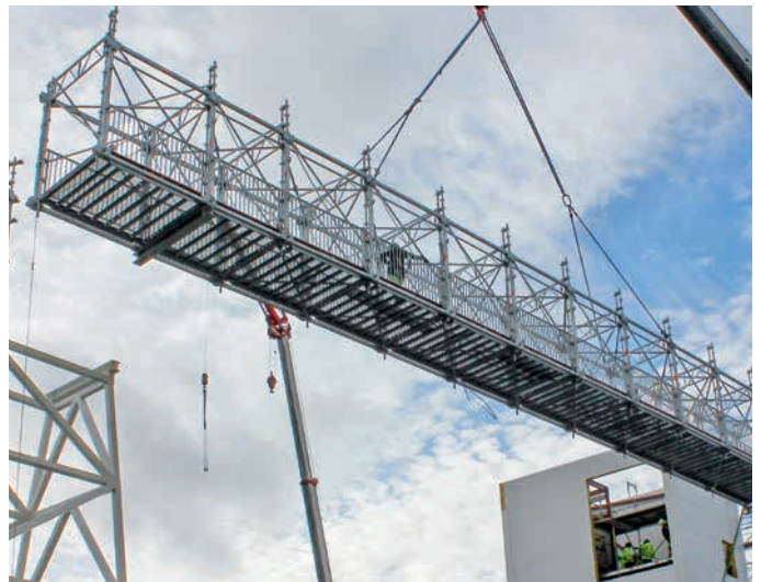
Footbridge preassembled on the ground with Allround Bridging System during crane positioning
