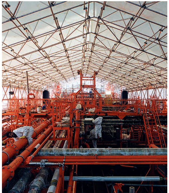
Keder Roof during maintenance of an oil tanker
