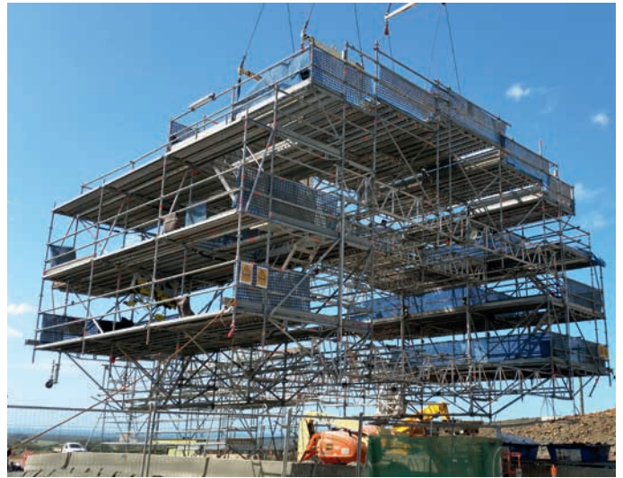
Rail-mounted mobile work scaffolding during crane movement
