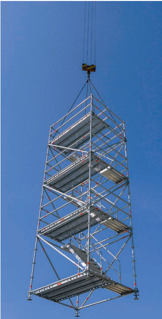
Unidirectional Allround modular stairtower during crane emplacement
