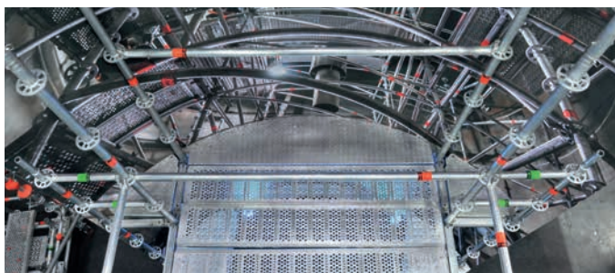
Round decks for scaffolding inside boilers
