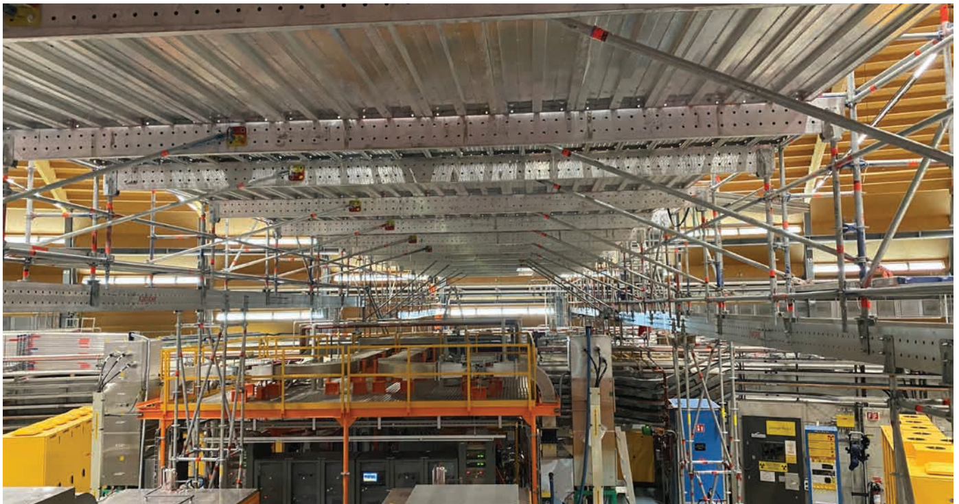
Wide-span ceiling scaffolding in an industrial hall while the facilities continue to operate
