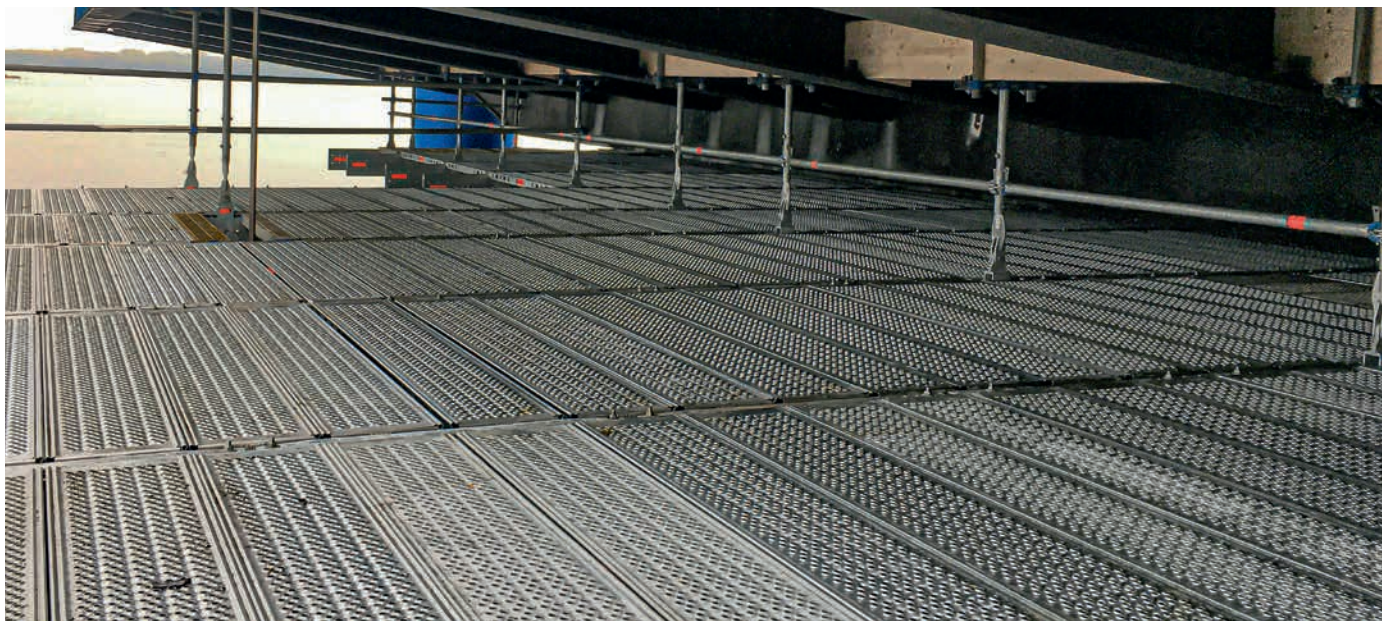
Non-trip and closed decking with standard steel decks
