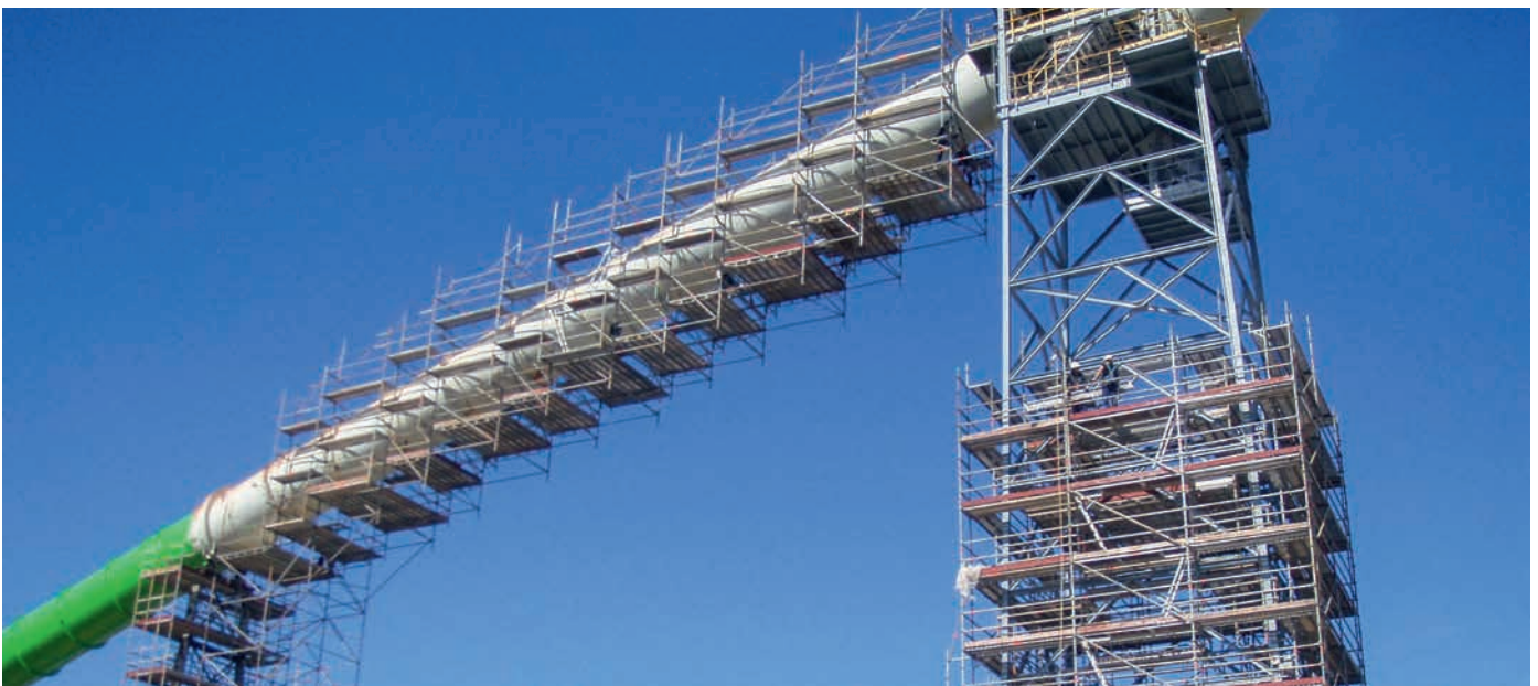
Suspended scaffolding structure on pipeline
